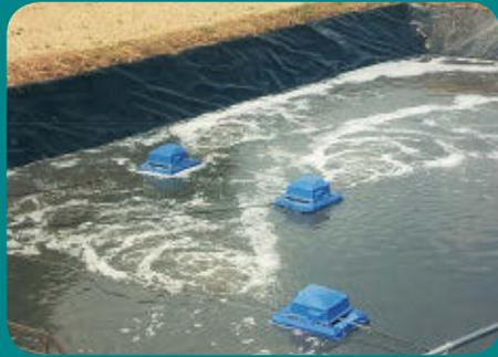
Turbo-Jet 1.1kW - three aerators working in an oxidation pond
